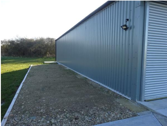
Potential location for fuel tank.
