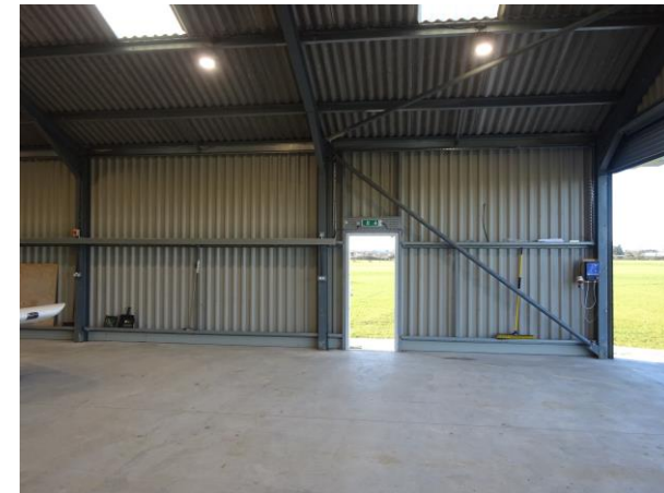
Side exit door/means of escape when front hangar doors are closed.
